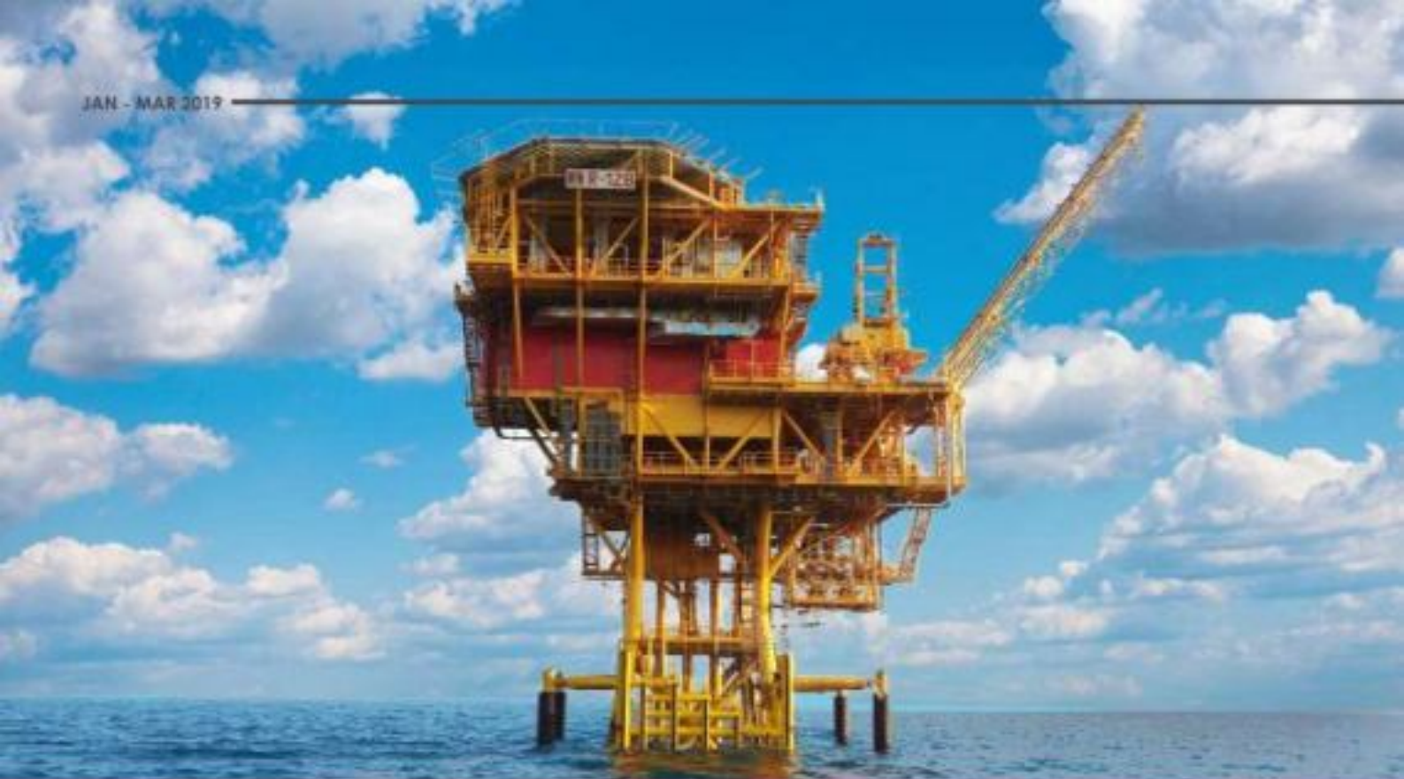
Oil & Gas Plant (Mumbai - Offshore)
