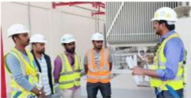
Work at Height - Al Murah South S/S
