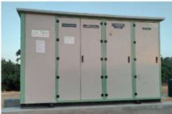
Minaran panels are successfully installed at 2x660MW STPP Udangudi site.
