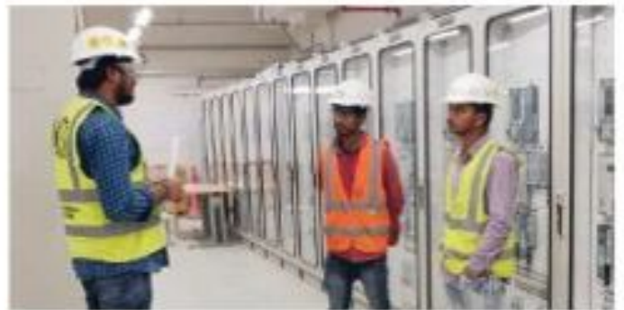
Importance of Personal Protective Equipment's - Ain Ahamad S/S
