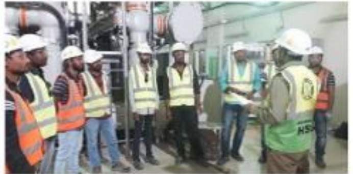
Doha Super Substation - Voltech Qatar
