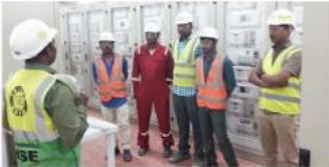
Lusail West-2 Substation - Voltech Qatar
