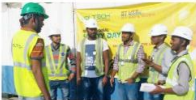
GE- HVDC- Kurushetra, ICD1 (HVDC)
